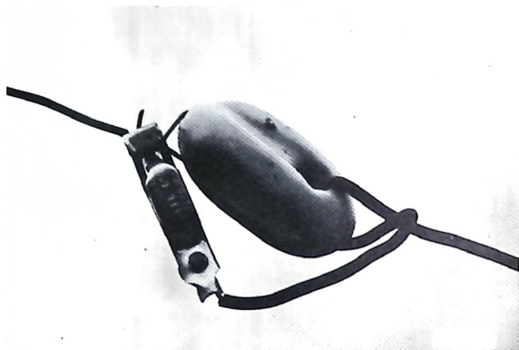
Fig. 8-8. Insulator and jumper.
