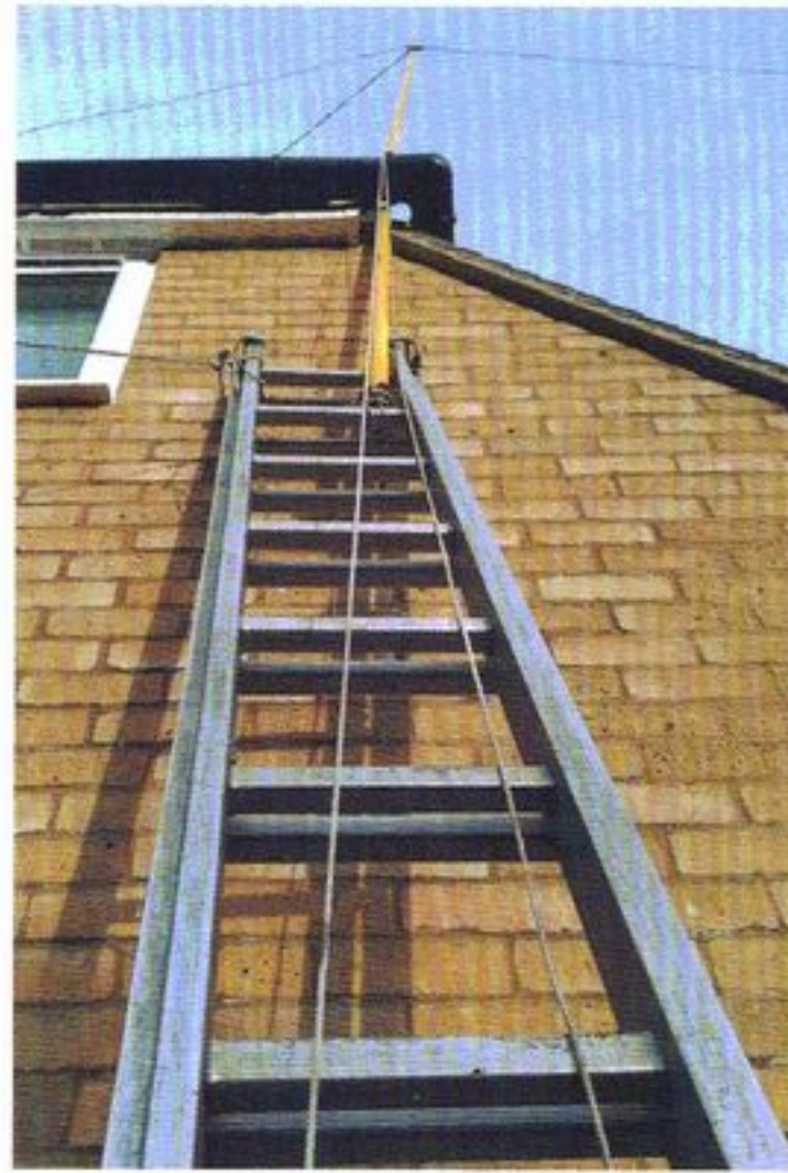
Looking up the ladder holding the fibreglass mast.
